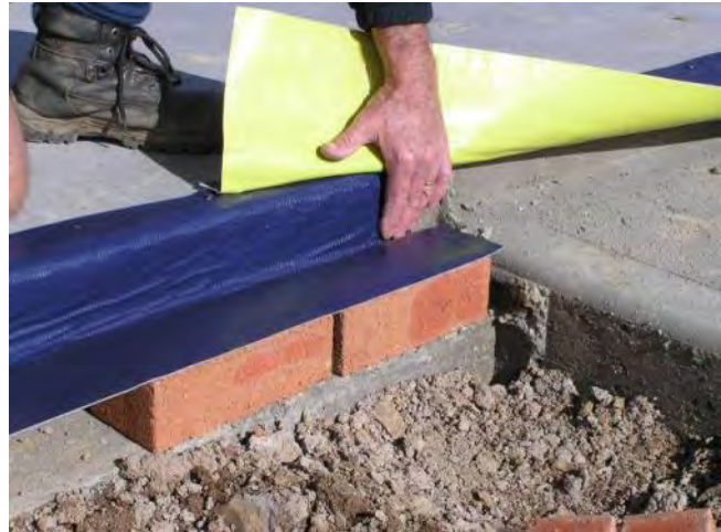
Lower strip of TRITHOR is pulled flush with face of bricks.
