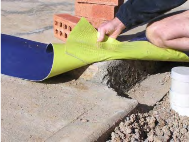
TRITHOR is left overlapped at corner
