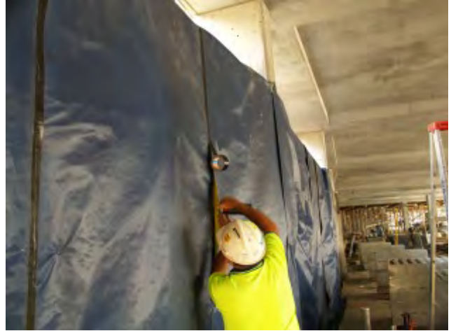
Apply glue to underside of top layer and attach to lower.
