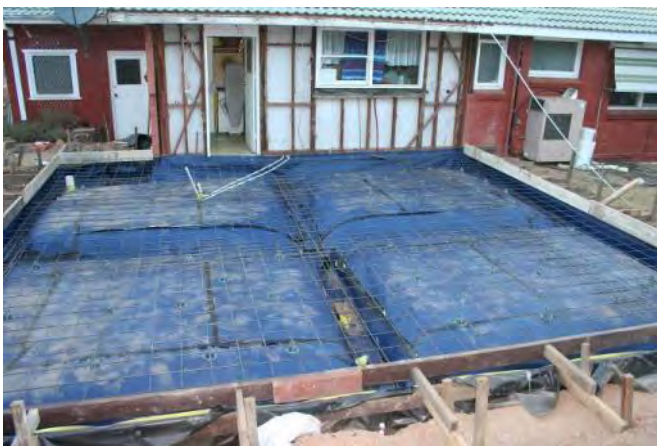
Figures 3 – 8 TRITHOR Termite Protection Plus NB Collars should not be taped as shown in Figures 3 and 4.
