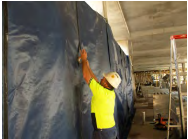
Apply tape over glue and press firmly to seal.
