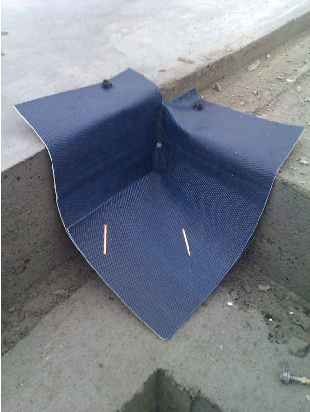
Figure 49 A Internal Corner
