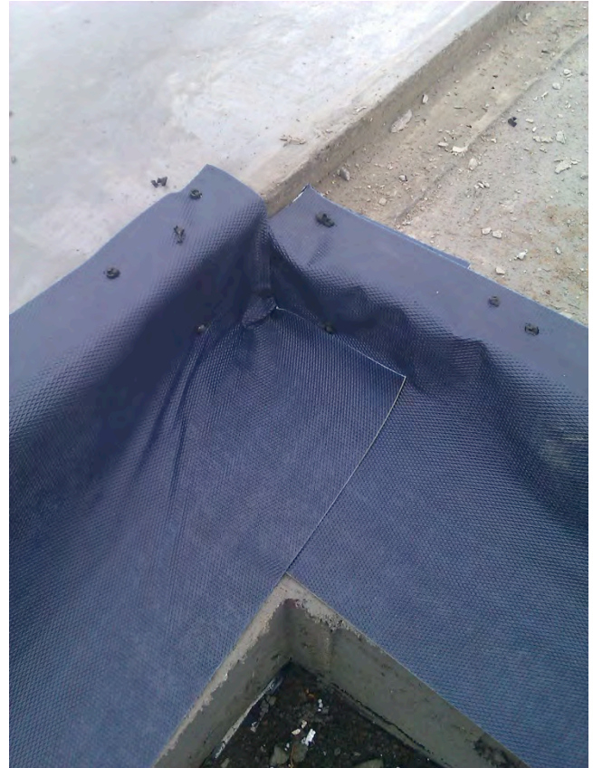
Figure 49 B Internal Corner with TRITHOR placed
