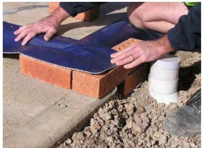
Upper strip of TRITHOR is laid over bricks on single brick transition and pulled flush to face of bricks on corner.
