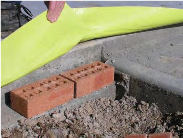
First layer of bricks are laid on rebate under TRITHOR.
