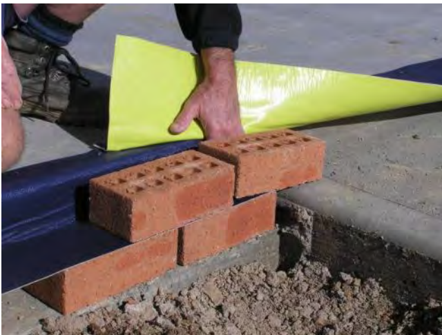
Second layer of bricks is laid over first strip of TRITHOR ensure TRITHOR edge remains flush with face of bricks.
