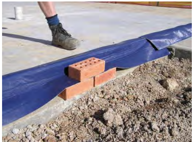
Second layer of bricks is laid ensuring TRITHOR remains flush with face of bricks.
