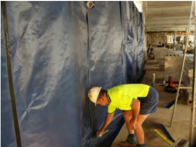
Apply glue to upper layer to give extra bond to tape.
