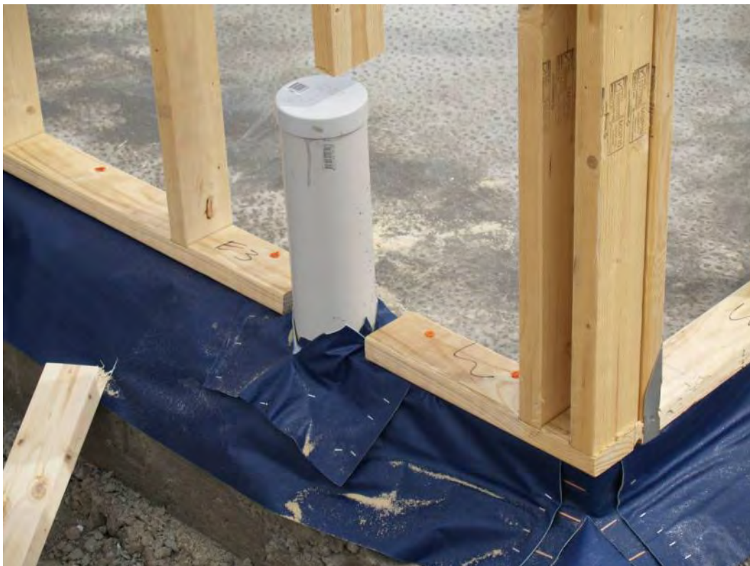
Figure 48 Two step rebate showing pipe penetration after frame erected.
