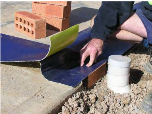
Lower strip of TRITHOR is pulled level with face of bricks with surplus pulled into cavity.
