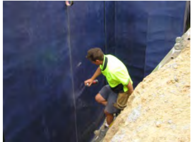
Apply further glue layer to outside
