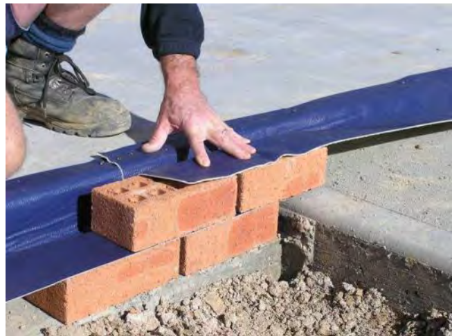
Top strip of TRITHOR is laid over second layer of bricks.
