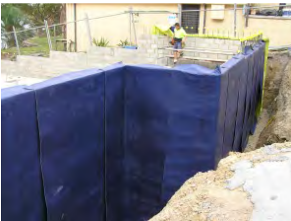
Install and overlap all sheets
