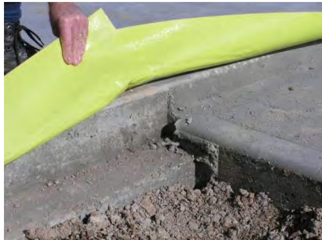
Lay first layer of bricks on rebate.
