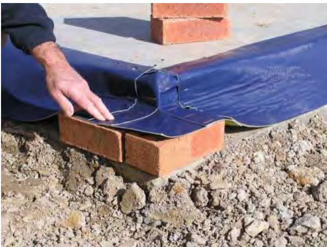
First layer of bricks is laid under TRITHOR with TRITHOR pulled level with face of bricks.
