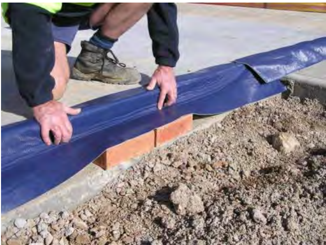
TRITHOR is pulled flush with face of bricks with surplus TRITHOR pushed into cavity.
