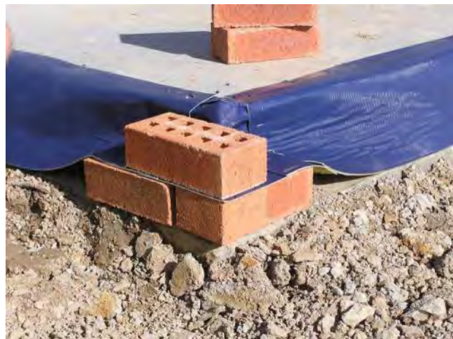
Second layer of bricks is laid ensuring TRITHOR edge remains flush with face of bricks.
