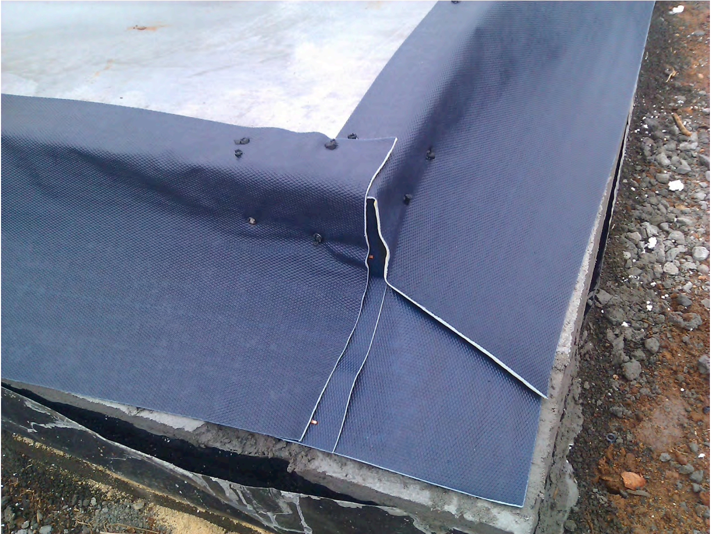
Figure 49 C External Corner
