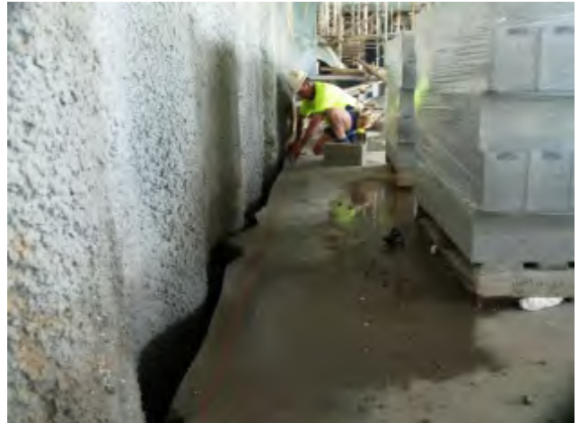
Use flick line to mark face of wall.
