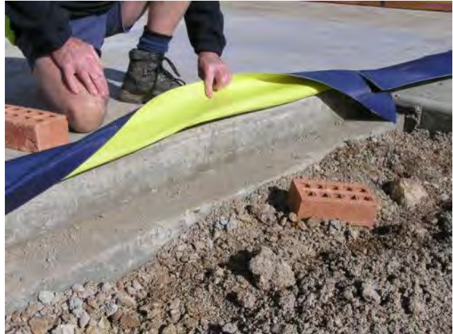
Lay first layer of bricks is laid on rebate under TRITHOR.
