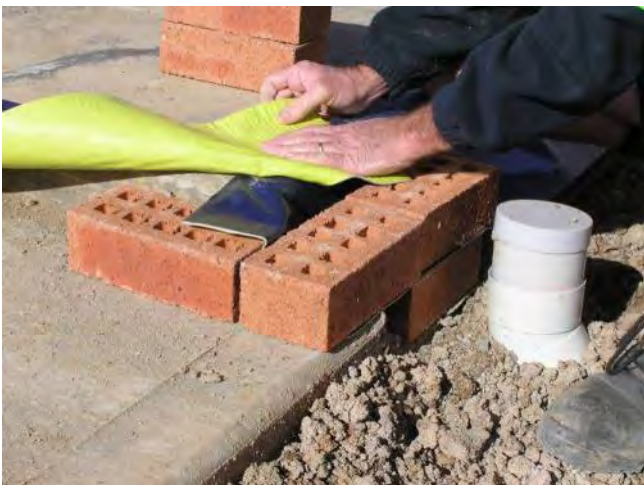
Lower strip of TRITHOR is pulled over first brick on single brick transition.
