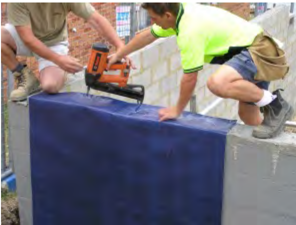
Secure with Ramset nails
