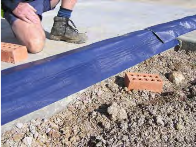
TRITHOR in position, nailed to slab.
