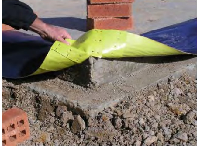
Lay first layer of bricks is laid on rebate.
