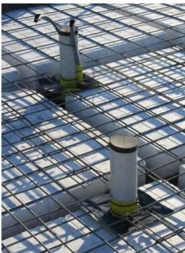
Figure 73 Pipe penetrations in waffle-pod slab.
