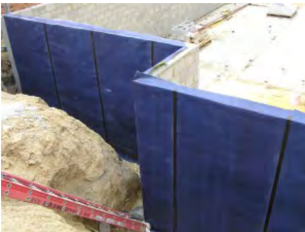
Retaining wall protected by TRITHOR
