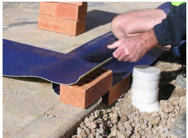
Second layer of bricks is laid over lower strip of TRITHOR and under upper strip of TRITHOR.
