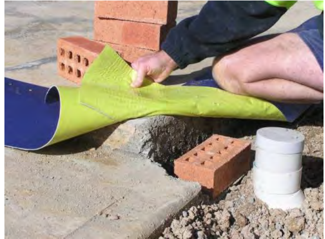
First layer of bricks is laid under TRITHOR.
