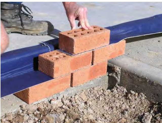
Next layer of bricks is laid.
