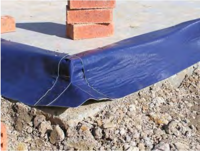
TRITHOR corners are nailed in position.
