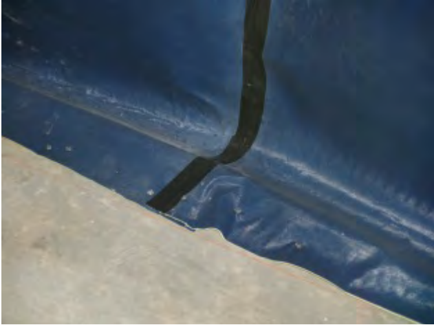
U shape ensures moisture behind the TRITHOR will run off and not 'wick' into the building in the future.
